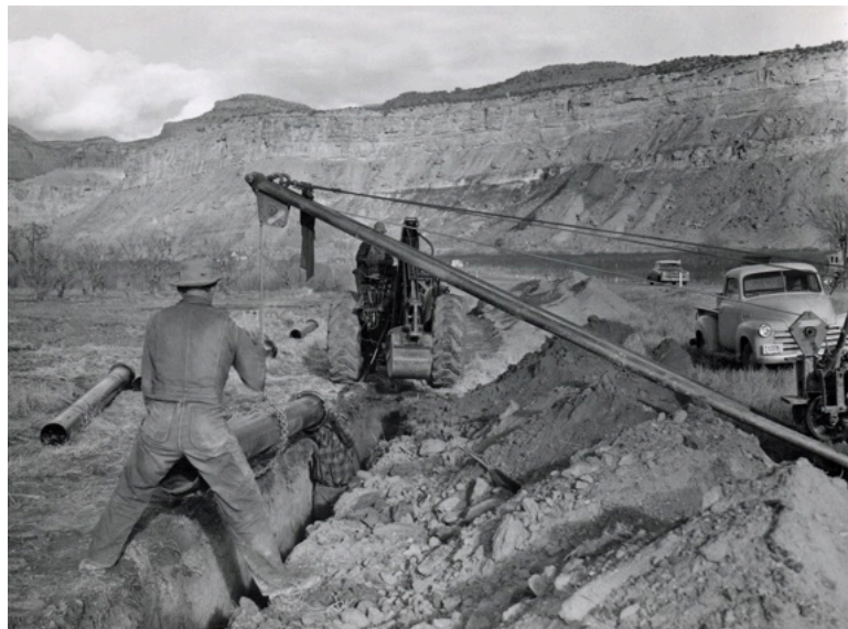
Laying municipal water pipes in the Vineland. (Photo courtesy of Jerry Nisbet.)
