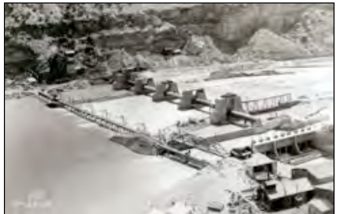
Rollers in Place — April 30, 1915.
