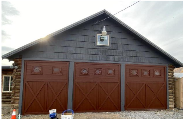
East side of the Bunte Shop painted March 16
