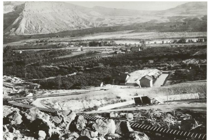
An early view of the Price-Stub pumping plant when it pumped water uphill into the Stub Ditch's wooden flume (lower right). Price Ditch water flows downhill into the canal just south and west of the pumping plant at this location. (Photo courtesy Orchard Mesa Irrigation District)
