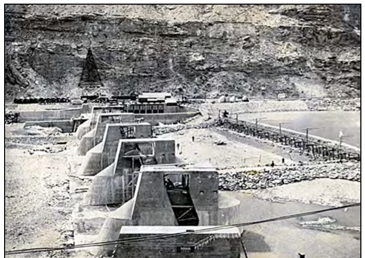
Roller Dam under construction in 1914-1915. (Photo courtesy of Robin Turcotte)
