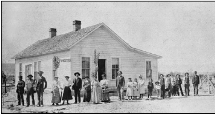
The Parton's house, hotel, and post office was located about where the Palisade Branch Library on 3rd street is currently. Courtesy of Museum of Western Colorado Palisade Library Collection.
